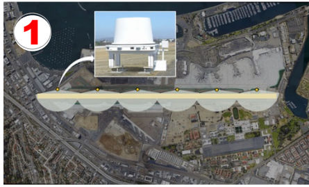
1 Radar units continuously scan 100% of runway surface.
